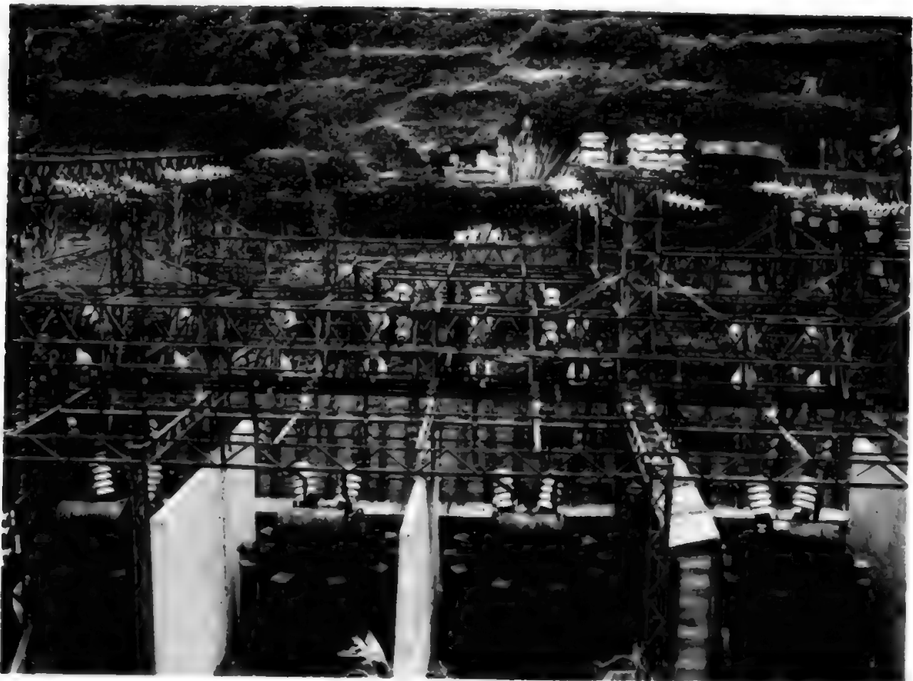
Figure 12.37b. Reinforced-concrete blast walls protecting transformers (1 mile from ground zero at Nagasaki).
